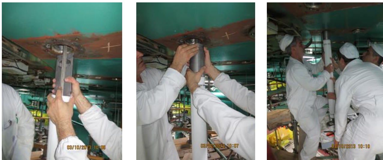
Figure 12. Mounting of the plugs at the bottom of IC channels on Unit 5.
